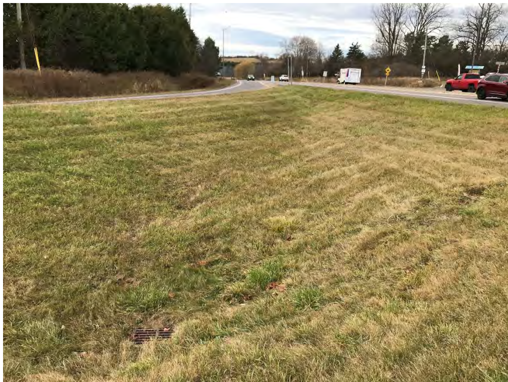
Photo 19 – Culvert CV-0007-005674 looking south – Nov 19, 2024.
