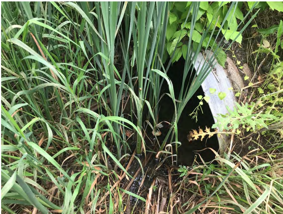
Photo 29 – Culvert CV-0007-000782 looking west – June 21, 2024.
