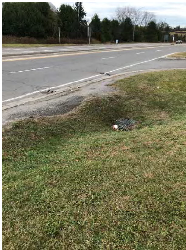
Photo 21 – Culvert CV-0007-005675 looking south – Nov 19, 2024.
