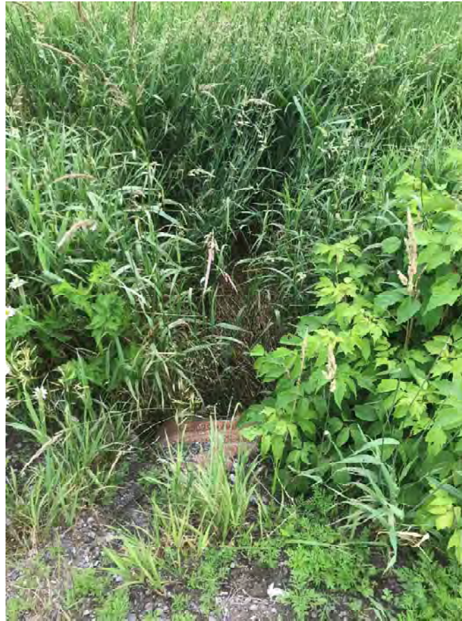
Photo 30 – Culvert CV-0007-000782 looking east – June 21, 2024.
