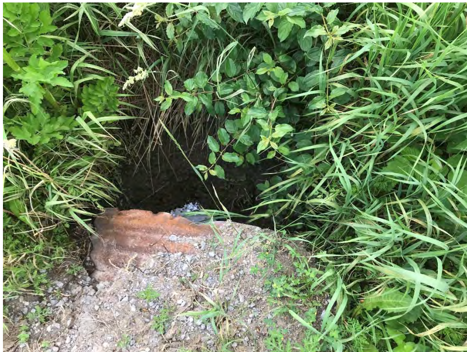
Photo 25 – Culvert CV-0007-000967 looking east – June 21, 2024.
