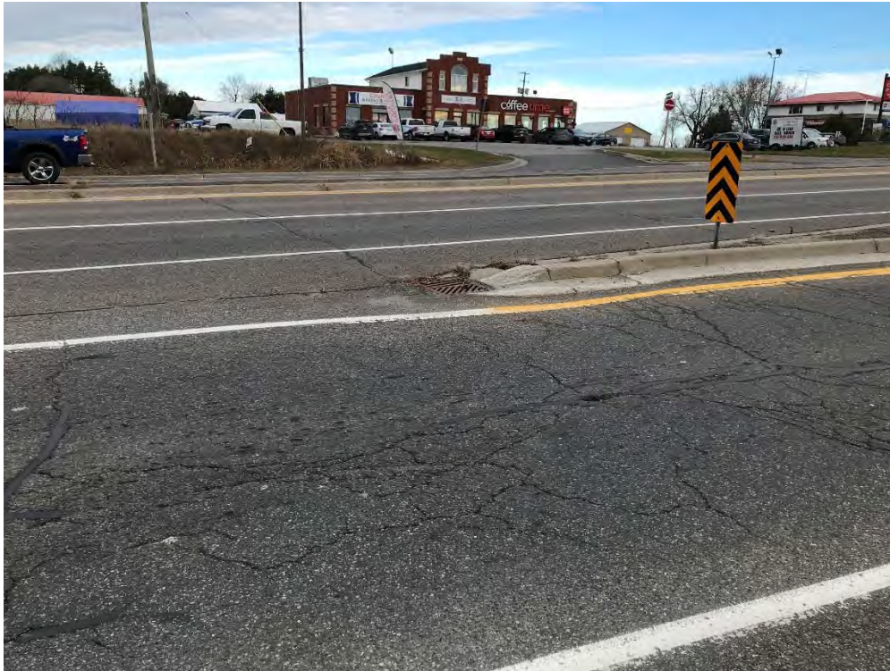
Photo 20 – Culvert CV-0007-000965 looking north – Nov 19, 2024.
