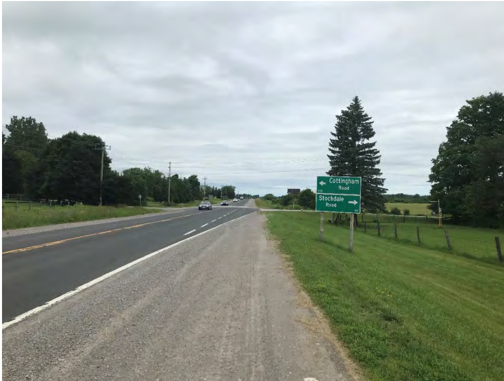
Photo 38 – Northbound lane view of Stockdale Intersection– June 21, 2024.
