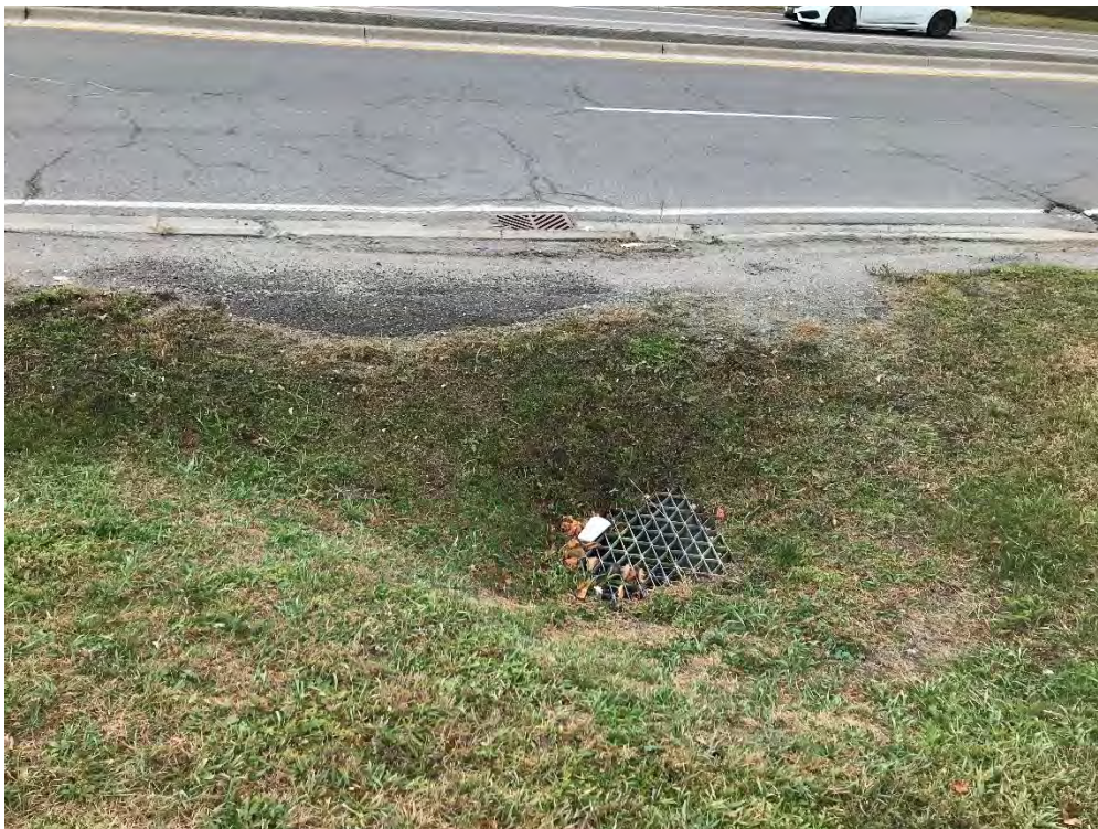
Photo 23 – Culvert CV-0007-005678 looking north – Nov 19, 2024.
