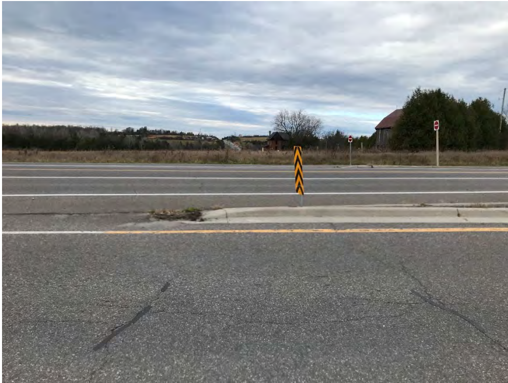
Photo 28 – Culvert CV-0007-000966 looking south – Nov 19, 2024.
