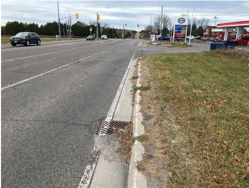
Photo 24 – Culvert CV-0007-005680 looking west – Nov 19, 2024.
