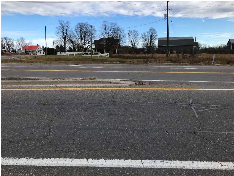
Photo 27 – Culvert CV-0007-005681 looking north – Nov 19, 2024.
