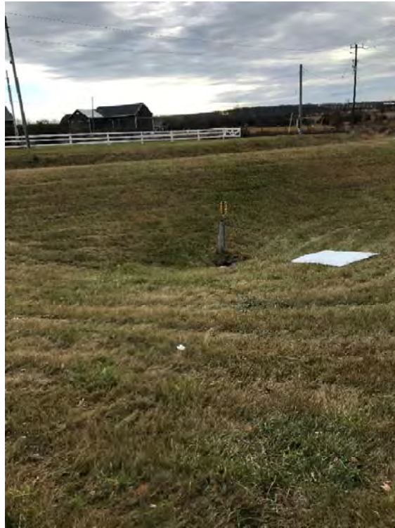
Photo 18 – Culvert CV-0007-000964 looking west – Nov 19, 2024.
