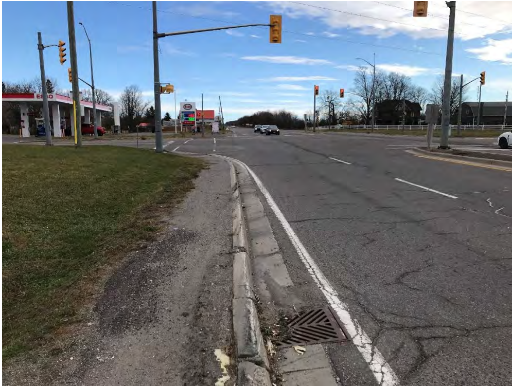
Photo 22 – Culvert CV-0007-005679 looking east – Nov 19, 2024.
