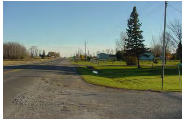
Plate 16: West side of ROW looking south at Cottingham Road.
