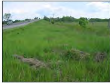
Plate 7: Looking south along the west side of the ROW at the disturbed area due to general road construction.
