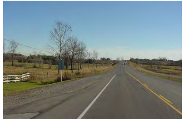
Plate 14: East side of ROW looking south with overpass in background.
