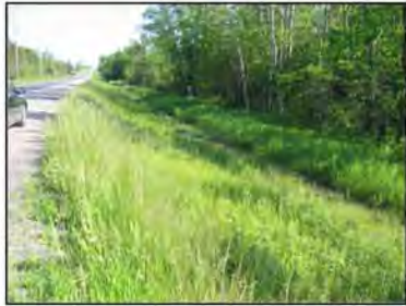
Plate 11: Looking north along the east side of the ROW at the ditch and the buried natural gas line.
